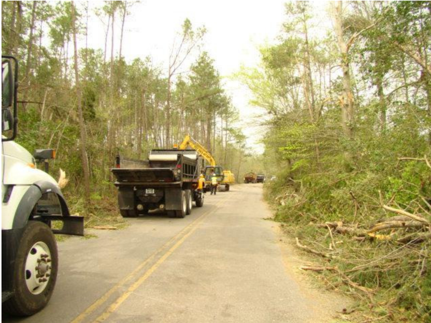
Debris Removal in Ware Neck Area of Gloucester
