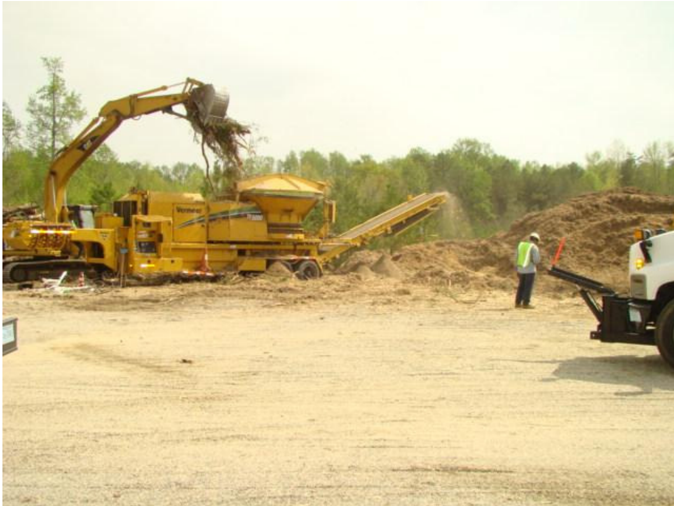
VDOT Debris Disposal Facility on Aberdeen Creek Road in Gloucester
