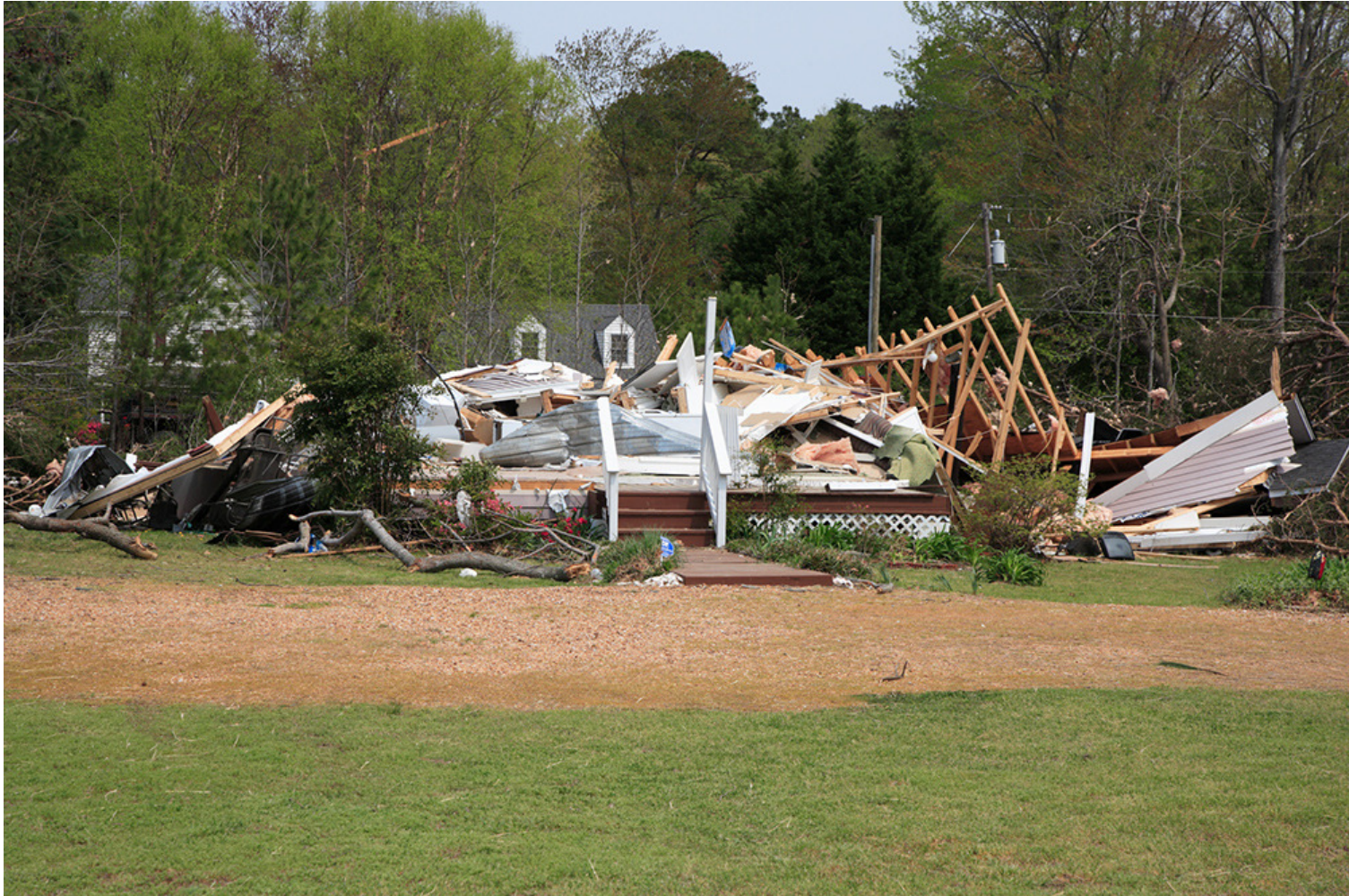
A destroyed home on Deagles Road in Deltaville
