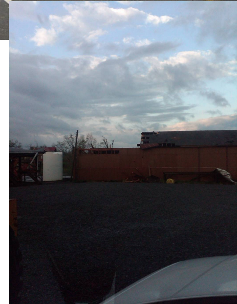
Signal and Sign Damage at Exit 29 & Route 11 Roof Damage at Glade AHQ
