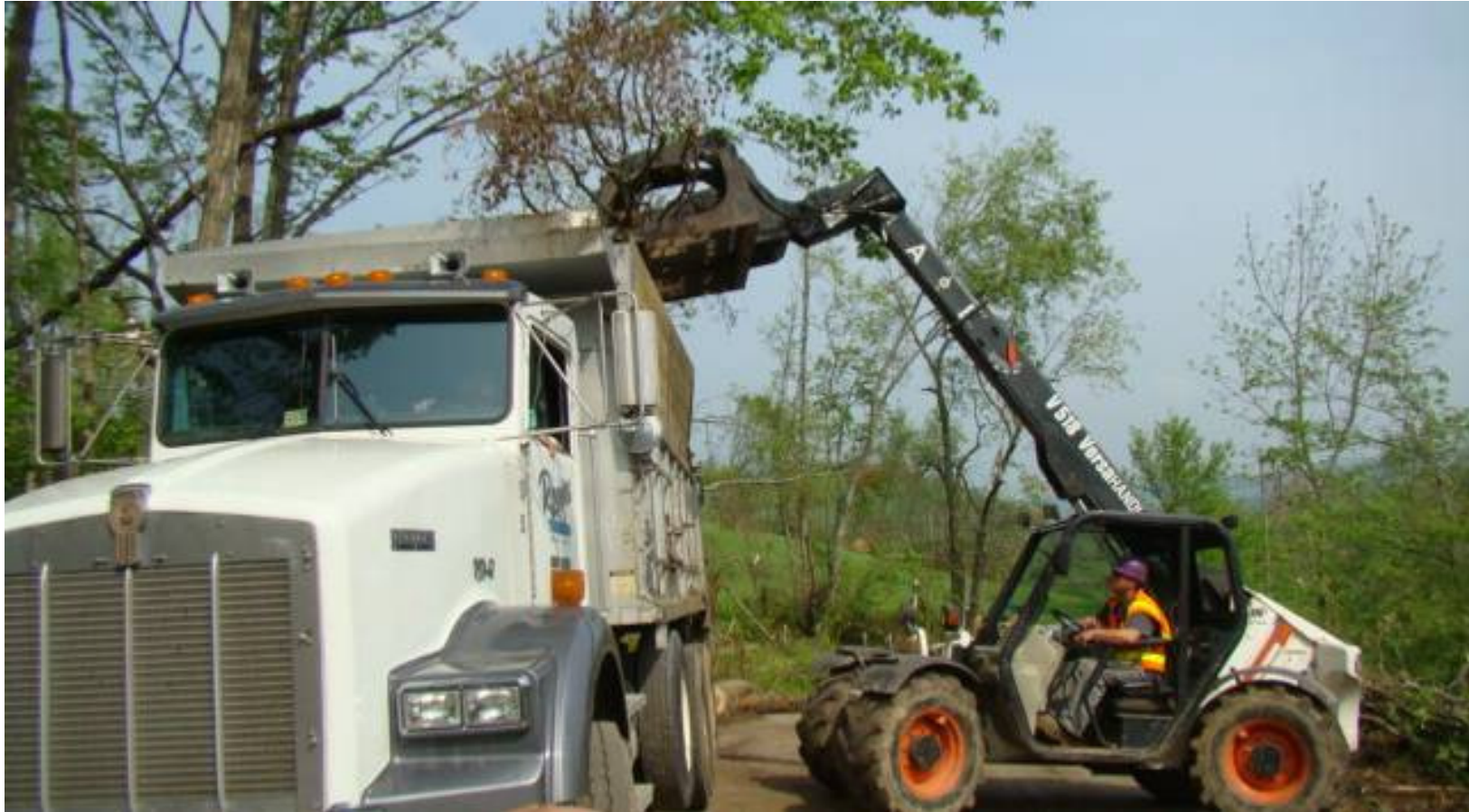
Debris Removal on Ramblewood Drive (Route 736)
