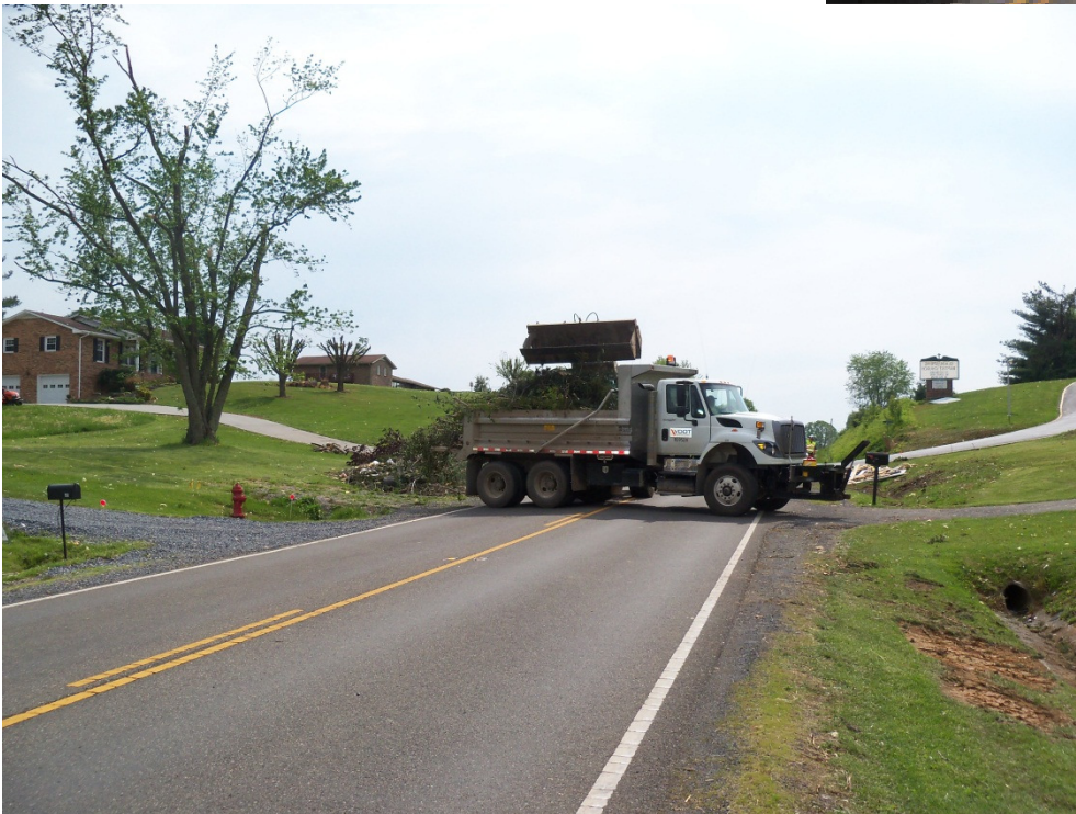
Debris Removal in Glade Spring
