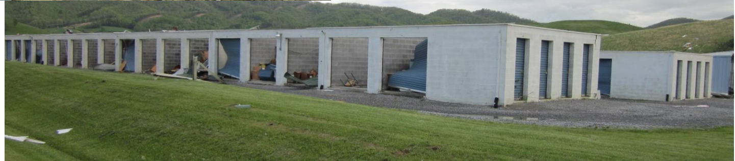
Damaged Businesses in Chilhowie
