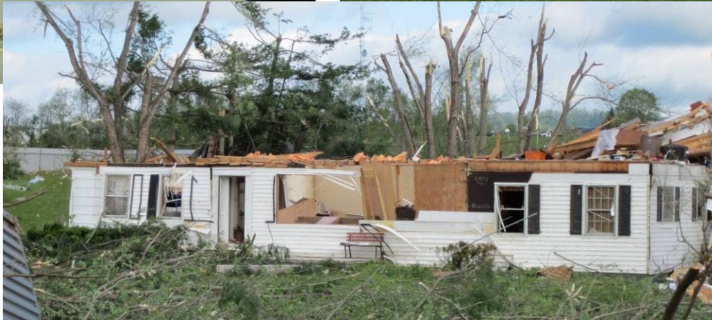
Destroyed homes along Route 11 North of Exit 29
