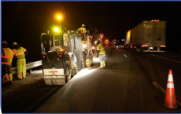
Mill and Overlay
