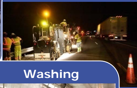
Mill and Overlay
