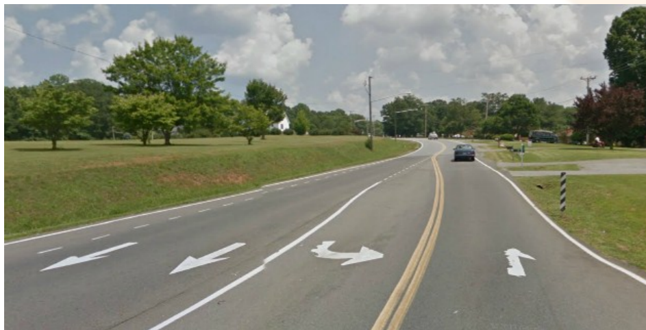
Widening Greenview Drive
