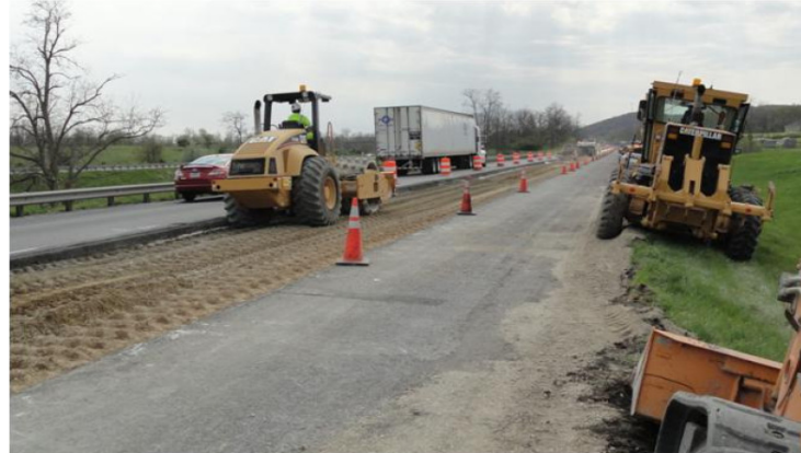
Full Depth Reclamation
