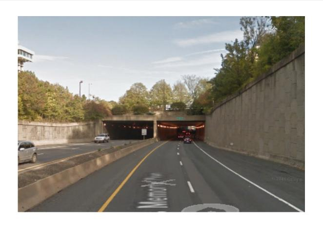
Deck over I-66 in Rosslyn and retaining walls constrain ability to widen I-66
