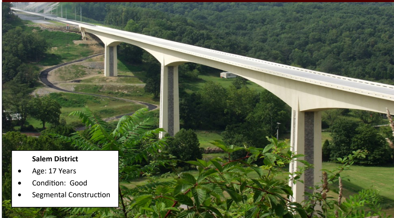
SMART Road Bridge (#17)
