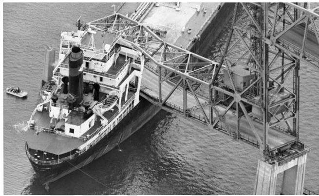
1977 Tanker Impact to Benjamin Harrison Bridge
