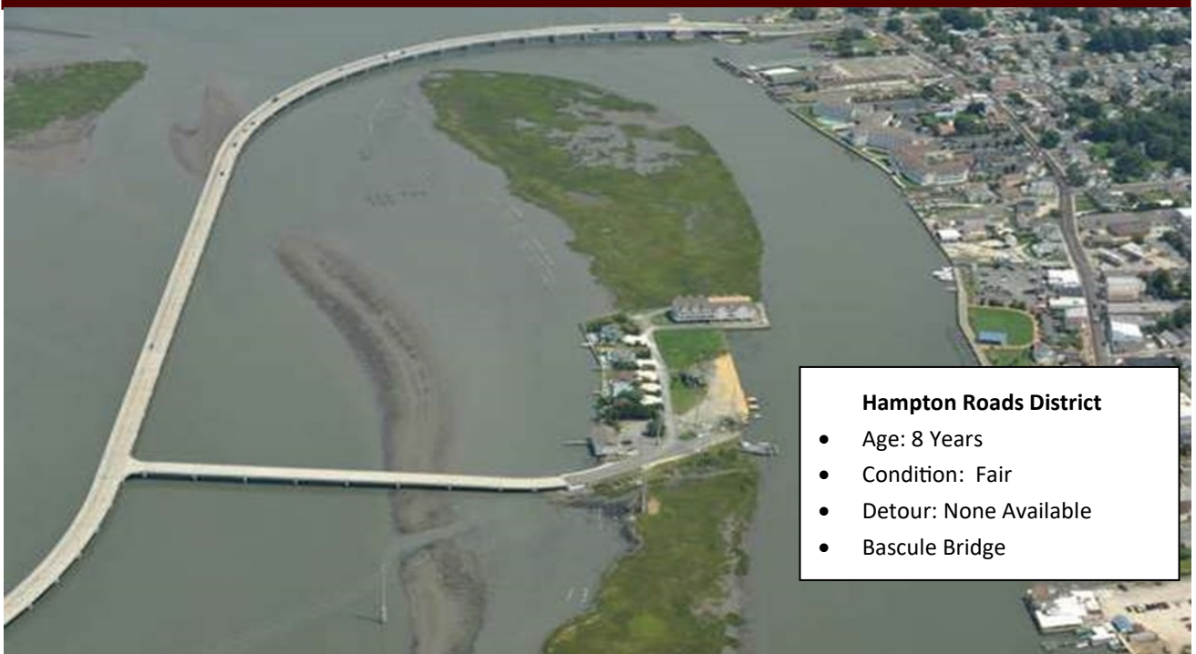
Chincoteague Bridge: Route 175 over Blackwater Channel (#2)
