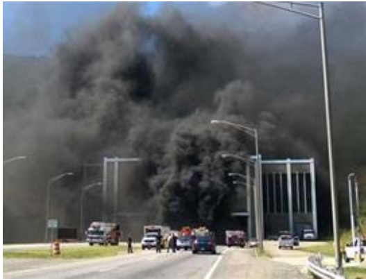
East River Tunnel Fire - July 2104
