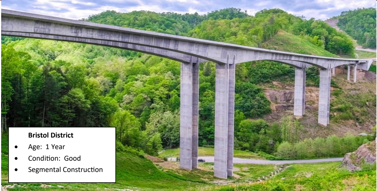
Route 460 over Grassy Creek (#16)
