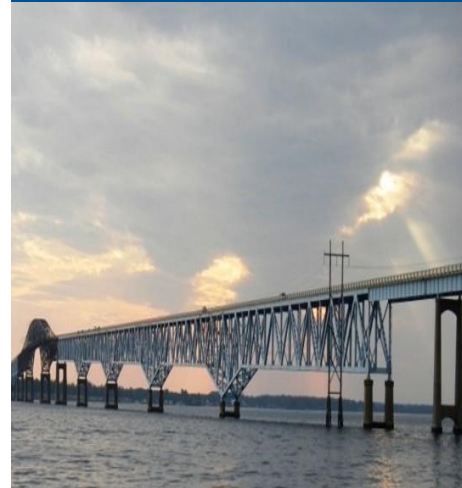
Robert O. Norris Bridge
