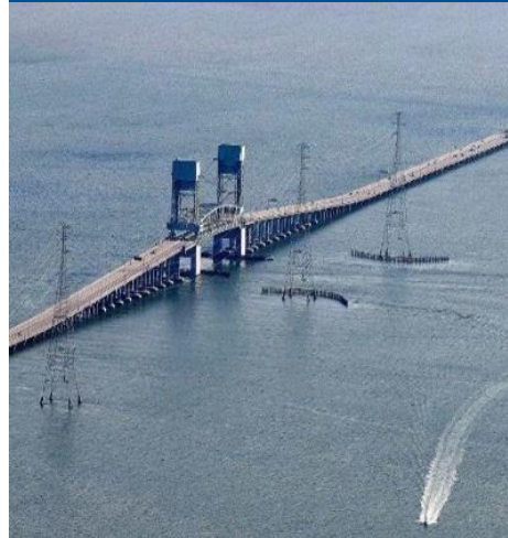
James River Bridge
