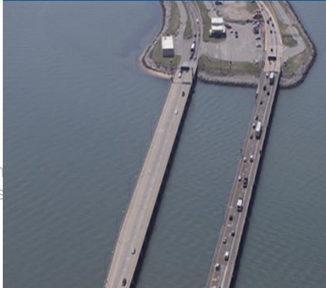
Hampton Roads Bridge-Tunnel Approach Bridges
