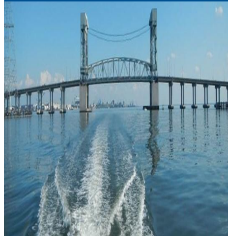
James River Bridge
