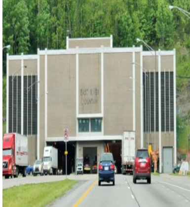
East River Mountain Tunnel
