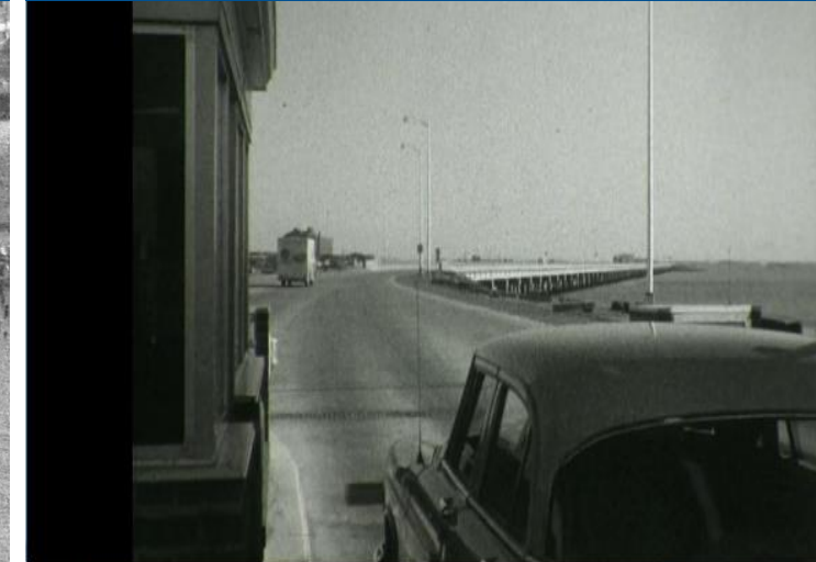
Hampton Roads Bridge-Tunnel
