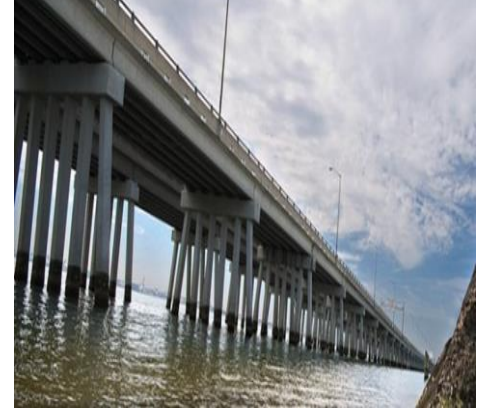
Hampton Road Bridge-Tunnel (Willoughby Bay)
