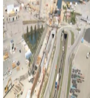
Elizabeth River Tunnel (Midtown)
