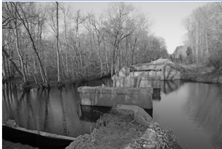
Carson Road (Rte 703) Bridge Replacement
