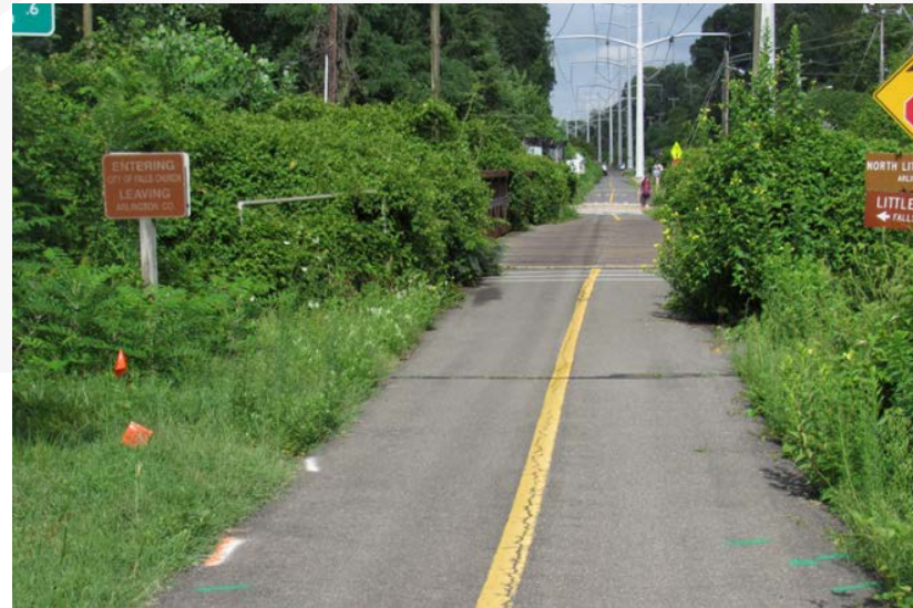
W&OD Trail, Falls Church Source: Toole Design Group
