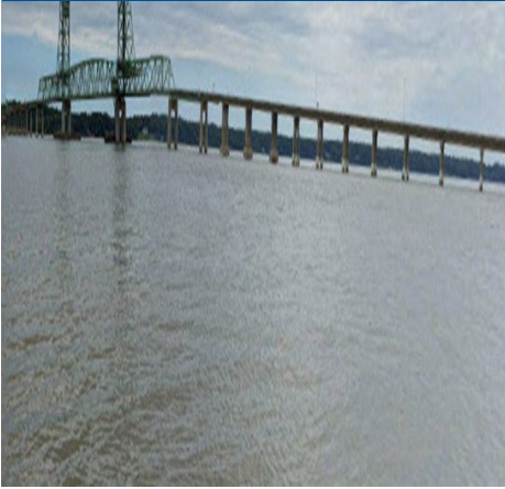
Benjamin Harrison Memorial Bridge
