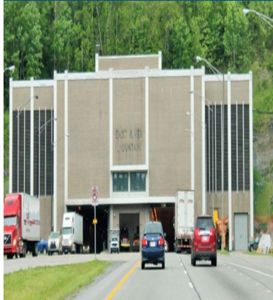
East River Mountain Tunnel
