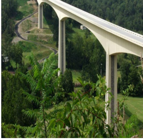
Gordon C. Willis SMART Road Bridge
