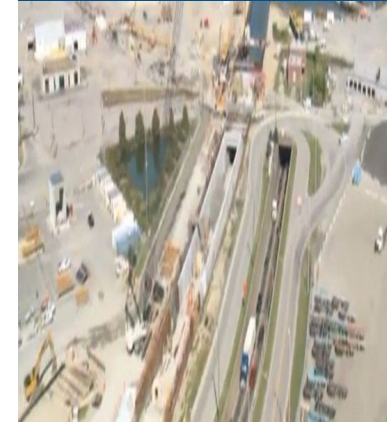
Elizabeth River Tunnel (Midtown)
