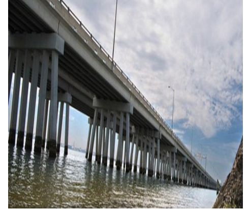
Hampton Road Bridge-Tunnel (Willoughby Bay)
