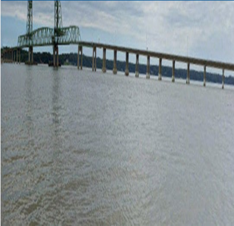
Benjamin Harrison Memorial Bridge
