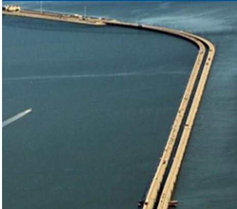
Monitor-Merrimac Memorial Bridge-Tunnel Approach Bridges
