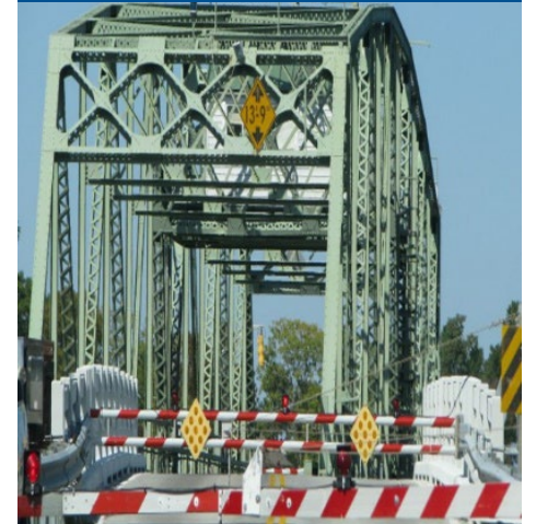
Gwynn's Island Bridge
