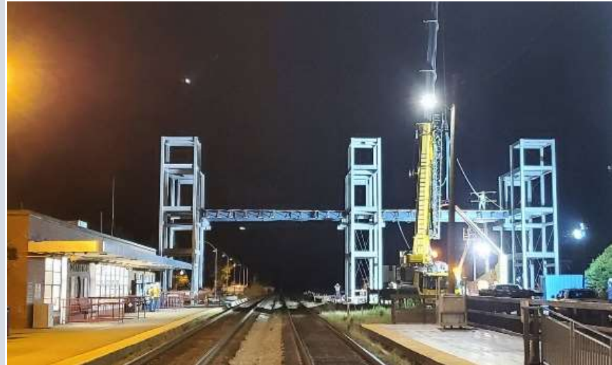
Pedestrian Bridge Construction at Quantico Station – August 2022.
