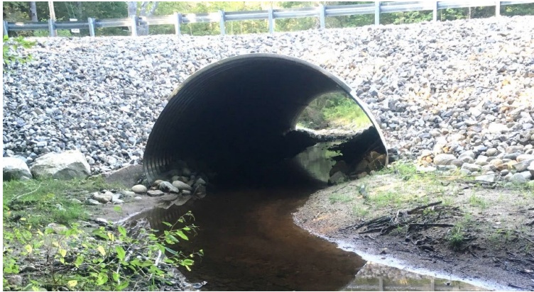
Corrugated metal arch pipe provides terrestrial and aquatic habitat values (USFWS).
