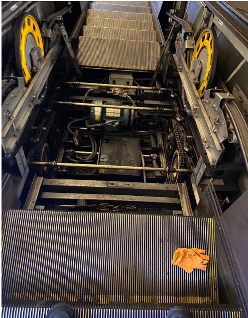
Escalator/Elevator Overhaul
