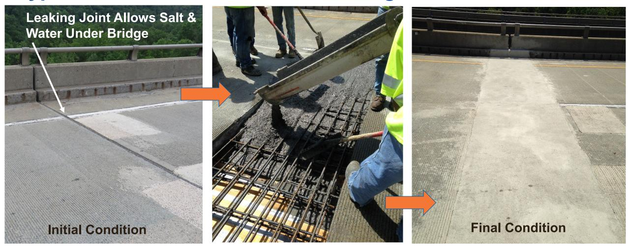
Protects Girders and Bridge Supports from Chlorides and Water 35 to 50 years additional service life for protected elements
