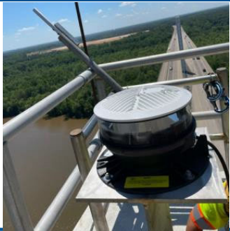
Installation of weather sensor
