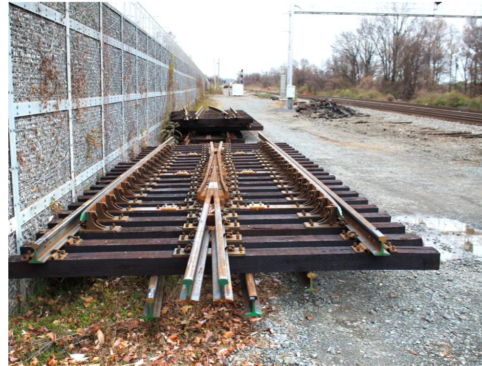
CSX is delivering materials on site
